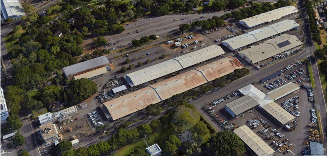
Figure 7. Existing Aerial View (Ameresco, 2023).
